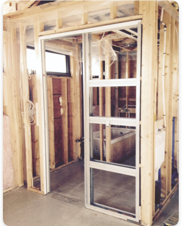
Mondoor metal pocket frame (satin coated steel 16 gauge) installed into wall. Pocket frame to be boarded vertically.
