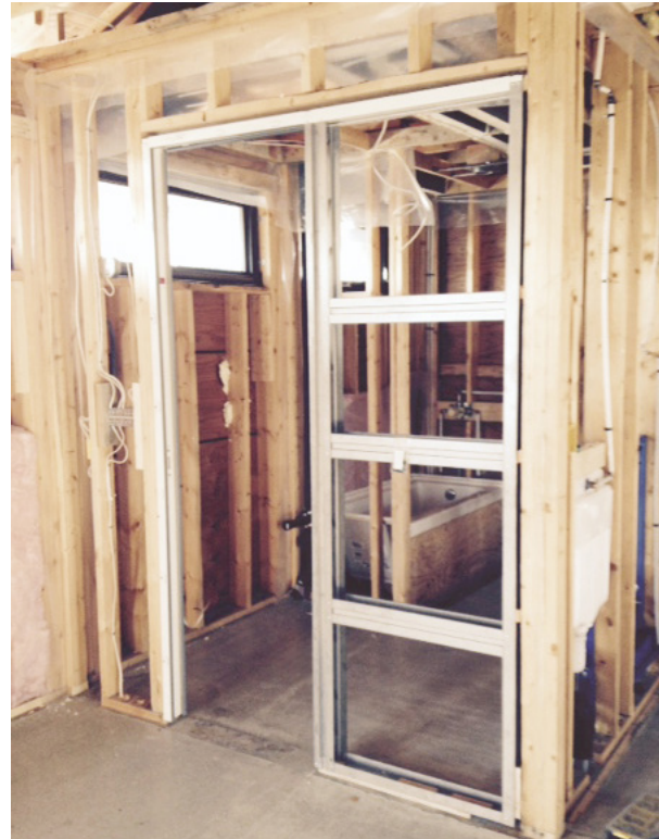
Mondoor metal pocket frame (satin coated steel 16 gauge) installed into wall. Pocket frame to be boarded vertically.
